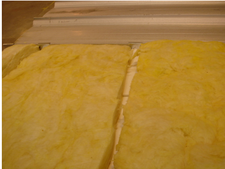
Fig. 2 Sag-and-Bag Configuration with Fiberglass Insulation
