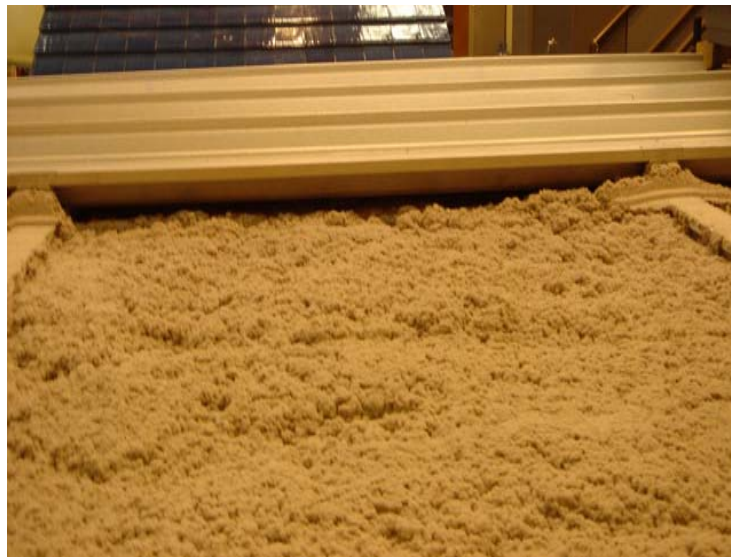
Fig. 1 Simple Saver Configuration with Cellulose Insulation
