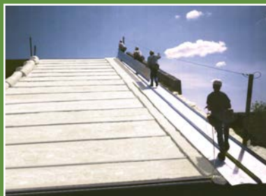
Install fiberglass insulation between and over purlins.
