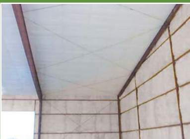
Fiberglass is full thickness and fills the girt depth.
