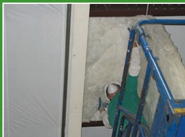
Pull or blow-in fiberglass insulation between the purlins.
