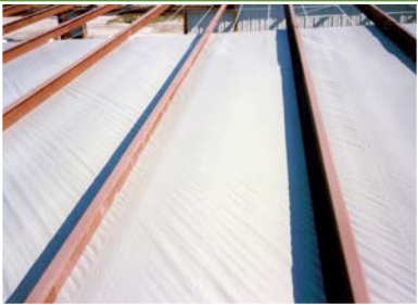
View of fabric liner positioned on strap platform and fastened to the structure.
