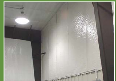
Finished wall and ceiling in manufacturing facility.
