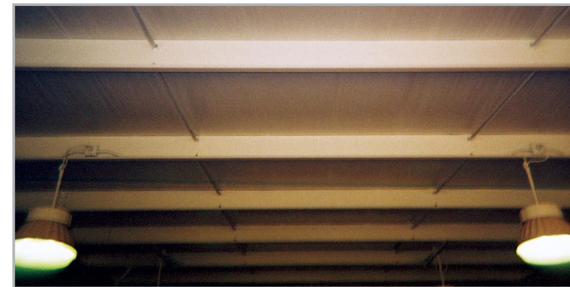
A typical over-the-purlin insulation installation photo, taken for a field measurement survey.
