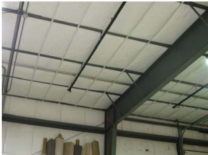
Liner System (top) and Filled Cavity (above)
